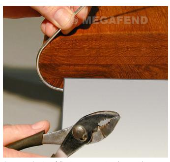
**Step 4**— Continue following contour using pliers as aid in bending rod to assure snug fit.
